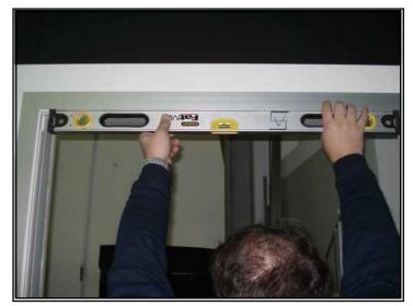
1.4.3 Tighten the screws permanently, cover the holes on the counterframe with the plugs supplied. The door is installed.Make a good cleaning (including removing the protective film from surface door) and applied the silicone to the external edges.Make a check on the correct gasket crushing as for attached table, which may regulate the striker for handle.
